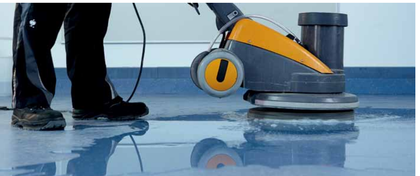
Repairing. Removal of stubborn dirt and scratches
