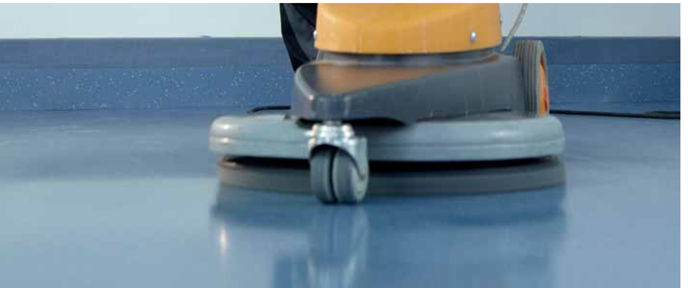
Finishing. First clean the floorings and polish them to a bright sheen
